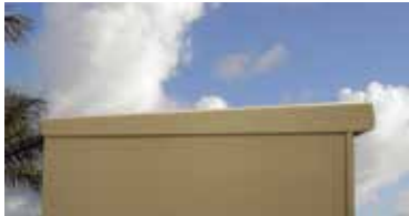
Sloped top for moisture runoff
